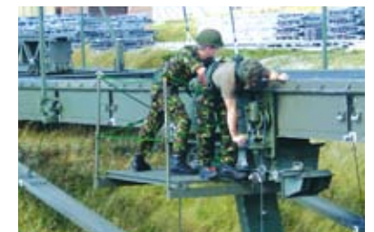
Top: An APFB Reinforced can span gaps of almost 30 metres. Middle: A DROPS Vehicle crosses an APFB Reinforced. Above: Tensioning the Reinforcement kit prior to crossing.
